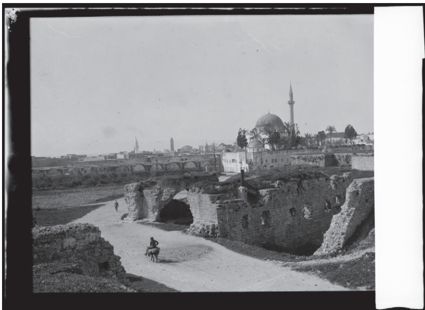
Fig. 8: "Tiberias seen from a distance," NINO, F. Scholten, Tiberiade , 20. A newly surfaced road into the city of Tiberias, running through the dilapidated walls and past a ruined fortress. The Great Mosque of Daher al-'Omar, now tragically neglected and used to store machinery by the Israeli municipality, stands proud in the distance.
