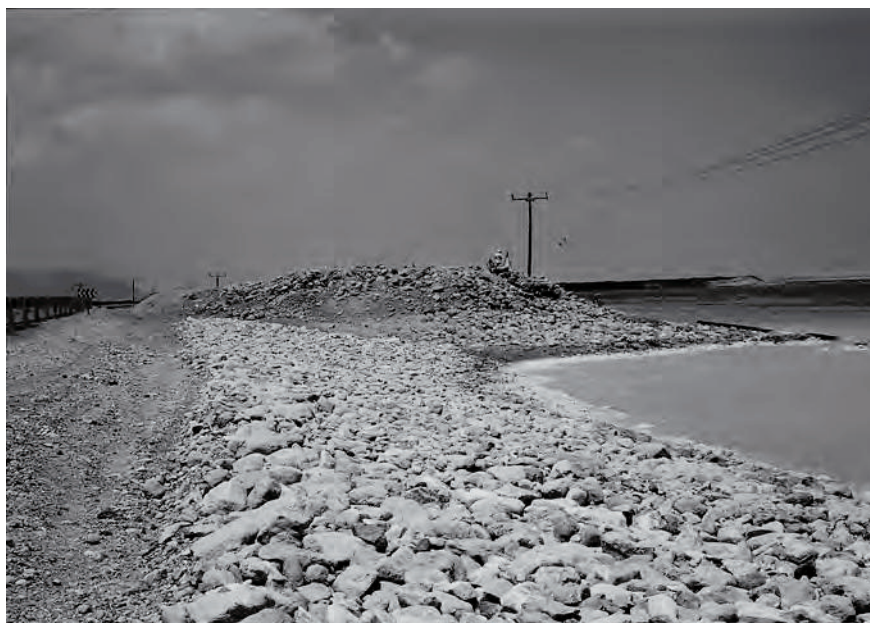
Figure 13.3: Mezad Gozal, looking north.
