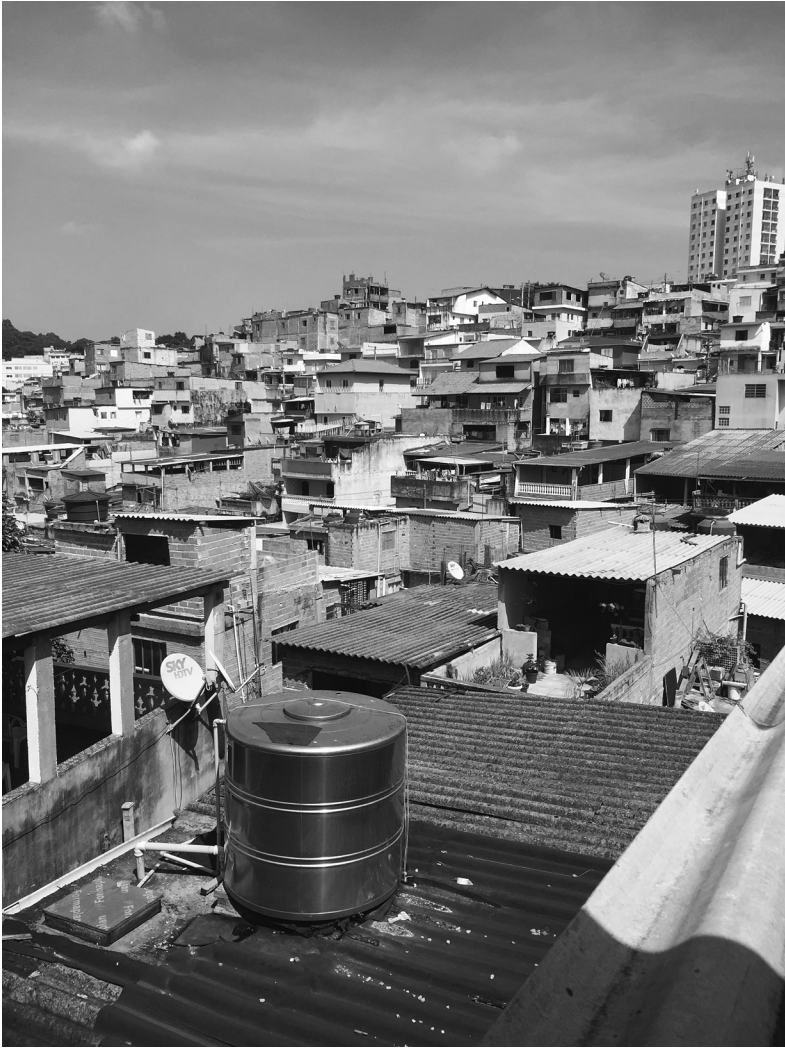
Figure 5.4 Water tanks on the roofs of homes in Capão Redondo, São Paulo, August 26, 2016. Source: Photograph by Jeffrey Lesser.
