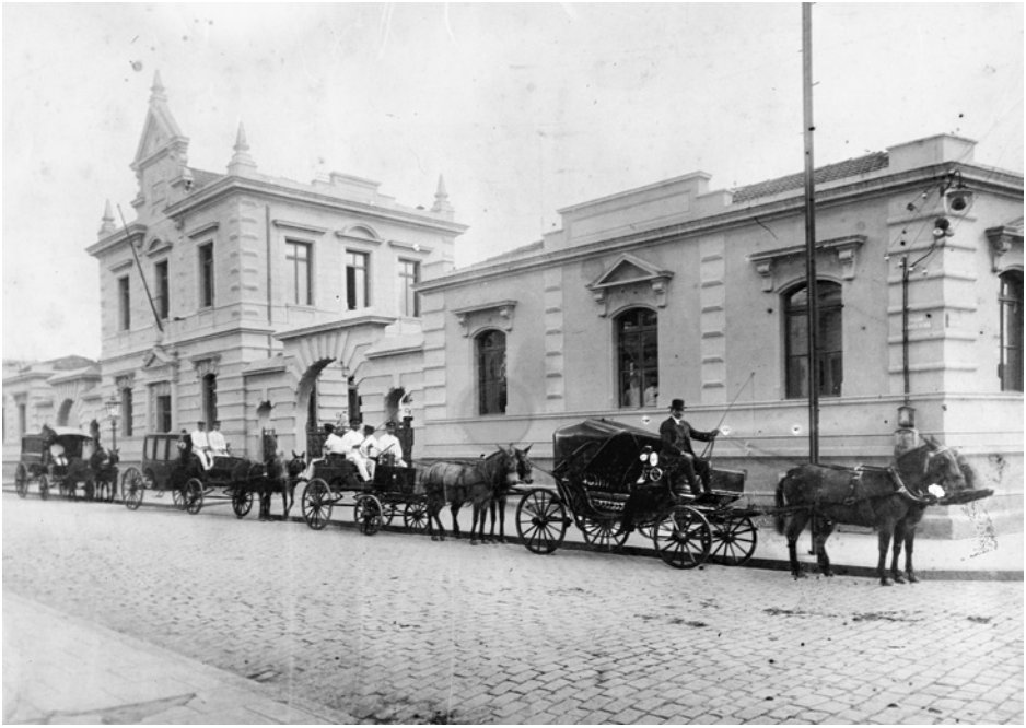
Figure 5.14 Facade of the Central Disinfectory with horse-drawn health service vehicles at the ready, ca. 1893. The vehicles have drivers whose white disinfection suits stand out visually. The vehicles are lined up in the following order: an elite passenger carriage, a transport vehicle filled with disinfectors, a people's passenger carriage, and a cadaver wagon. Source: Emílio Ribas Public Health Museum: Fachada do prédio do Desinfetório Central, R. Tenente Pena, Ampliação fotográfica, pb. [ca. 1893], Fundo Serviço Sanitário de São Paulo, Grupo: Desinfetório Central, Acervo Instituto Butantan/Museu de Saúde Pública Emílio Ribas.
