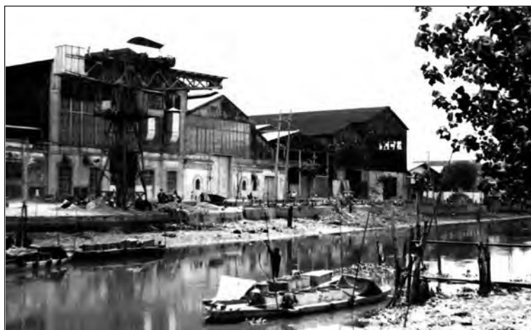
Figure 5.1. The old engineering workshop “de Industrie” on the east bank of the Kali Mas in 1987, shortly before demolition. Note the heavy crane. Photo by author.
