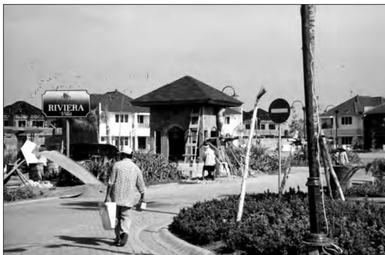
Figure 6.9. Gated community under construction, Laguna Indah, 1997. Photo by author.
