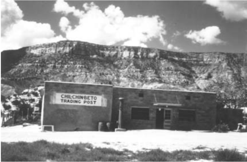
Chilchinbeto Trading Post in 1956. The left side of the structure was the original post, while the right side is an addition made in 1944. Behind the post sits Black Mountain. (Photo by Joe C. Hunt)
