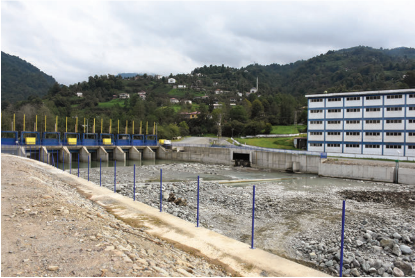
Figure 5.9. The blue-and-yellow structure on the Orçi River is the HEPP construction. The riverbed is occupied by concrete, stones, and rubble, sparking protests in 2015. Arhavi, September 1, 2018. Photo by author.
